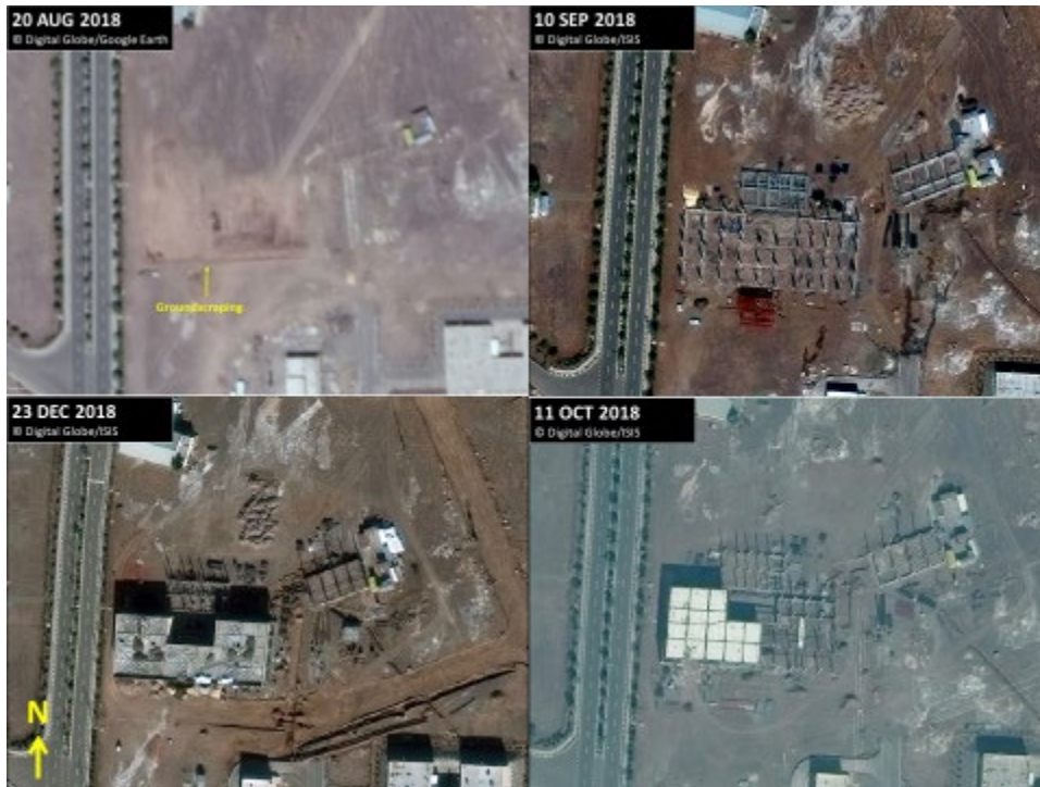
Figure 4.4. Construction timeline of the Vacuum Center, clockwise from upper left.
